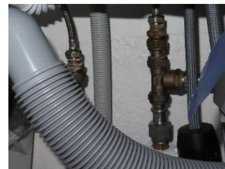
Messingfitting i rustfri installation
